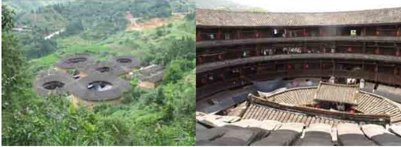
Figure 8. Tulou buildings/Roof details, Fujian Province. Photos by the author; (Left) External, (Right) Internal
